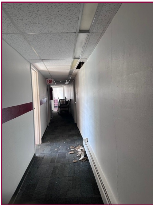
Hallway Inside Pressbox
