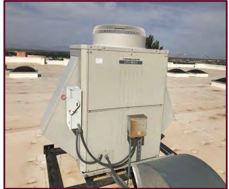
VRF Condensing Unit On Roof
