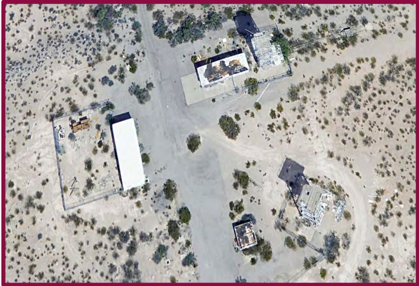
Communication Tower Site
