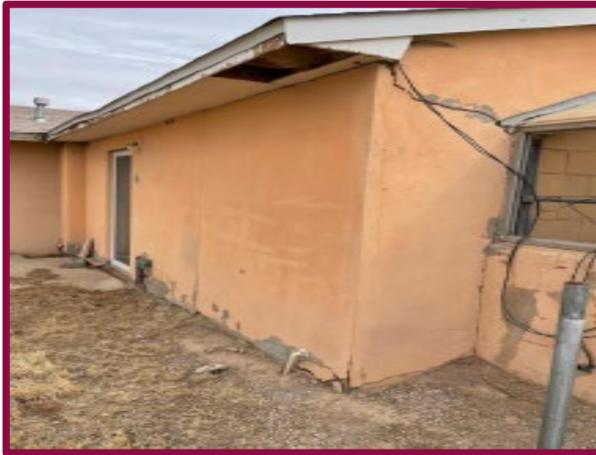
Exterior Settlement on Foundation & Roofline
