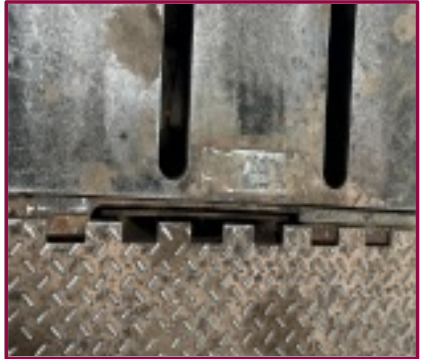
Automotive Shop Spill Containment Floor Drain
