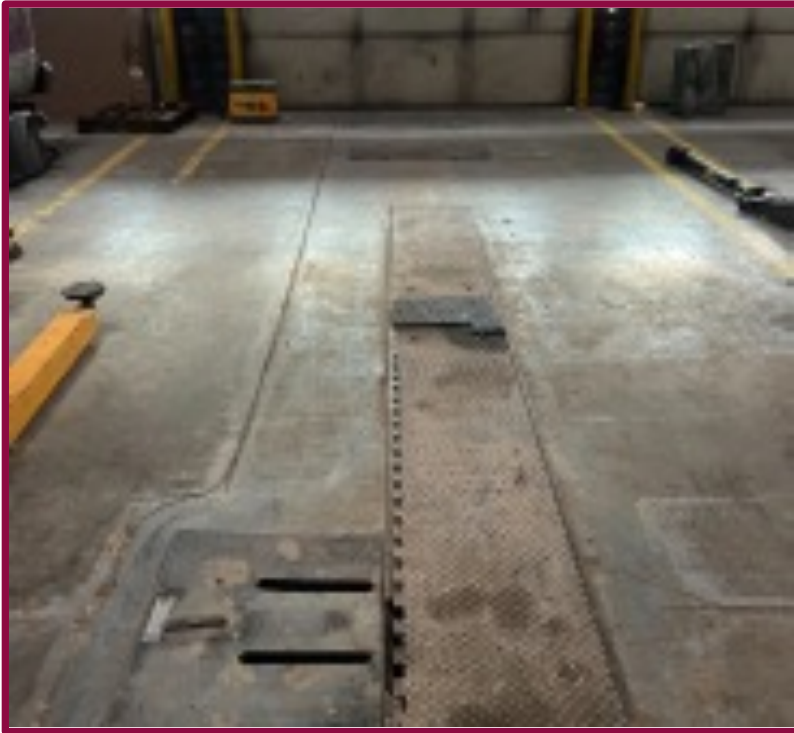
Automotive Shop Spill Containment Floor Drain
