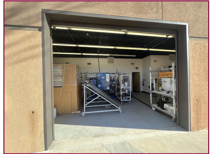
Existing Lab from Exterior of Building
