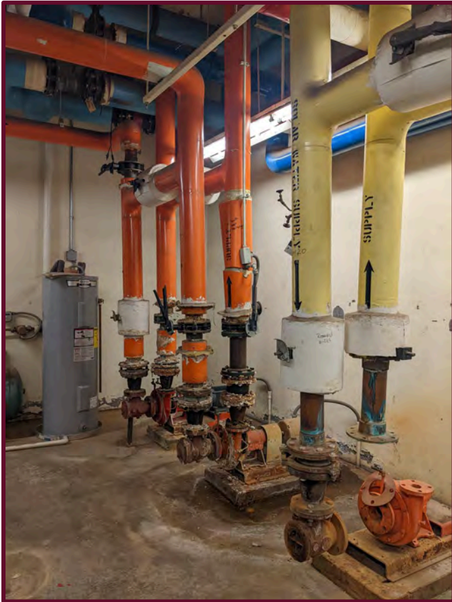
Chilled water utility infrastructure to be removed
