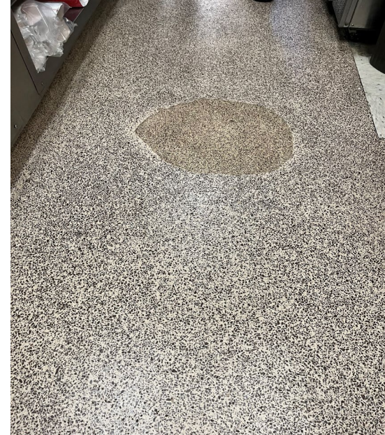
Flooring is aged and becoming more porous. The deterioration of the flooring is a New Mexico Environment Department violation and can be a fire violation as well due to the concrete absorbing grease.
