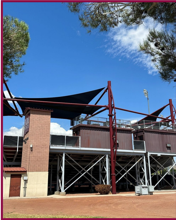
Wind damaged sails and cabling system
