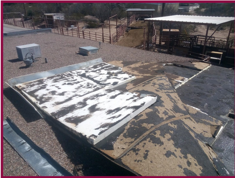
Wind and rain damage
