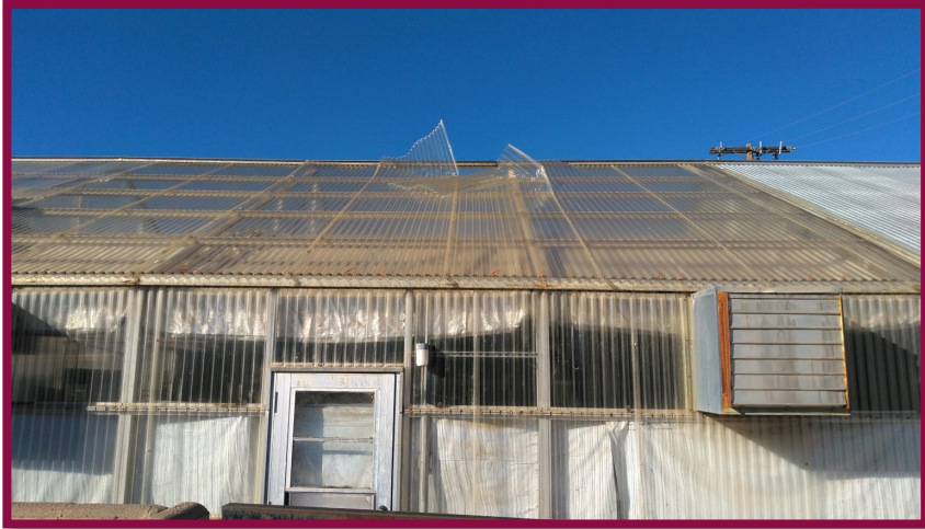
Wind damaged roof panels and ridge cap
