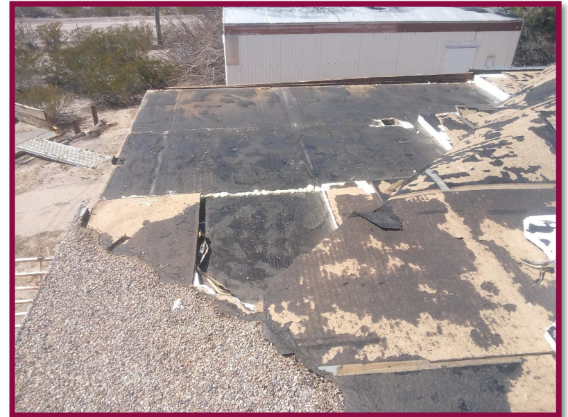
Wind and rain damage
